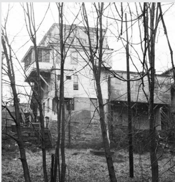
The town's renewal consultants found that most of the buildings in Moodus Village were substandard. One reason is that structures in the business district rested on tall foundations built of wood or cinder block along the bank of the Moodus River. Photo courtesy of Ken Simon.
