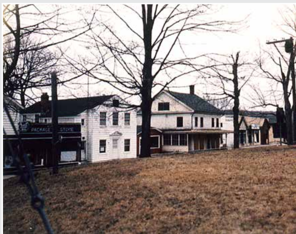
In 1967 the Moodus Center business district was emptied of its stores, offices and residences in preparation for demolition.
