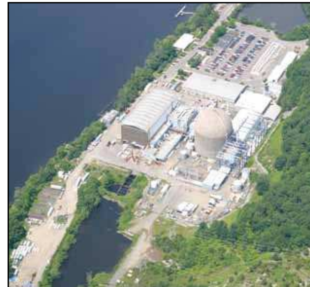
Connecticut Yankee in 2003, before major plant structures were demolished ( Connecticut Yankee, Haddam, Connecticut ).
