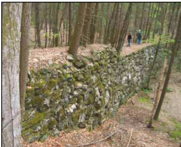
Left: the stonework for the dam at the millpond that supplied water power for several Haddam Neck millworks, particularly the paper mill on Pine Brook above. The paper mill was one of a series of mills in that building, including an earlier cotton mill and an oakum factory.
